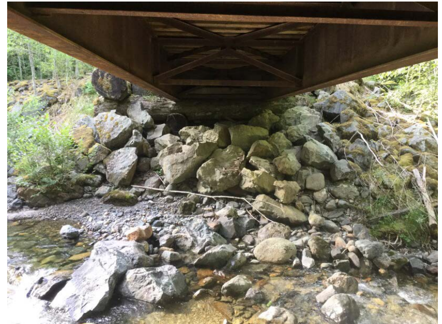
Left Bank Abutment when facing downstream
