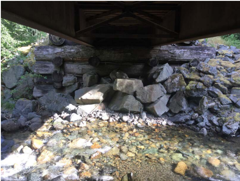
Right Bank Abutment when facing downstream
